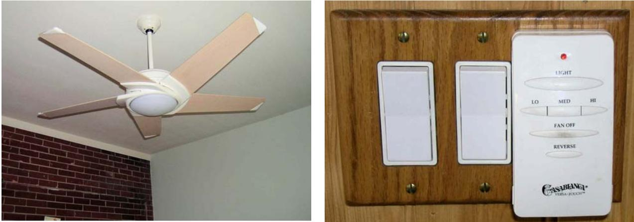
*Figure B-8. The controls for this fan allow for reversing flow and setting at three speeds.*
