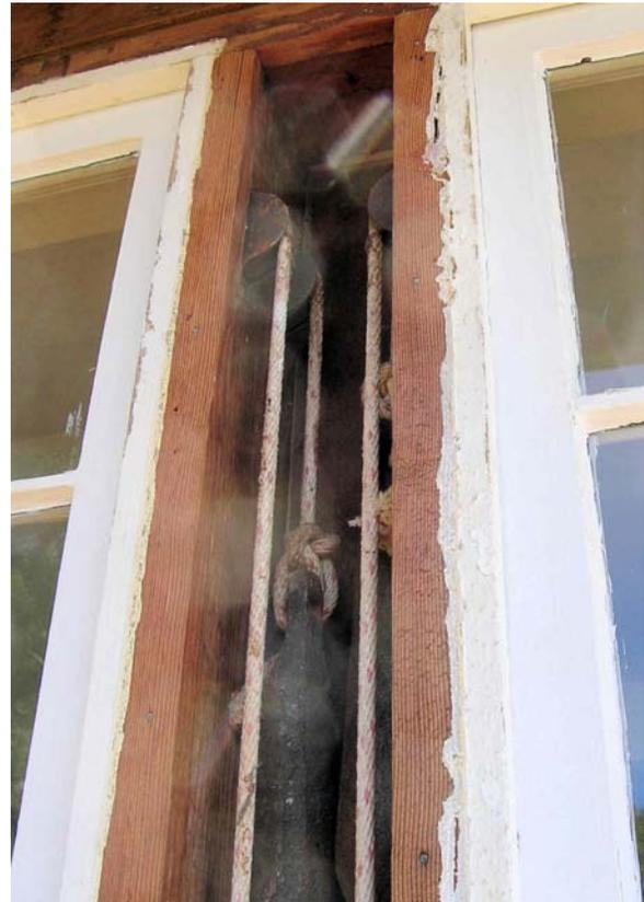
***Figures D-2 and D-3. An effective procedure for air sealing and insulating the weight box while retaining good functionality of the windows could be a useful retrofit for a wide range of windows in older homes. Assessing the practicality of the process and energy savings should be done well.***
