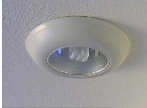
**Figure B-6. Installation complete. A thin bead of clear caulk (latex acrylic with silicone) was used at the interface of fixture and ceiling followed by a damp cloth. Then 12 inches of fiberglass was installed over the fixture, matching the other insulation in the attic.**
