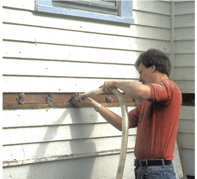
***Figure B-2. Drilling sidewalls and installing cellulose to high density using the tube method lowers both convective and conductive losses.***
