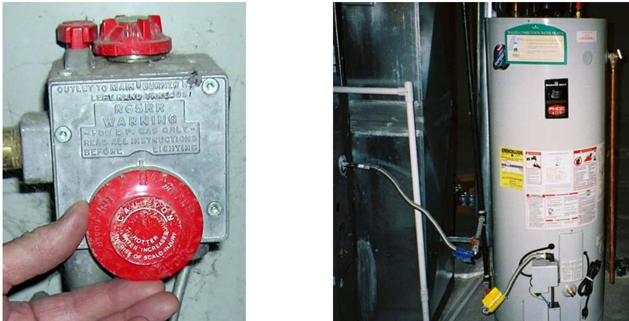
***Figure B-7. Adjustments of hot water heater thermostats need to be confirmed by measuring temperature at the sink. The heater on the right is much more efficient than conventional heaters because it is closed combustion.***
