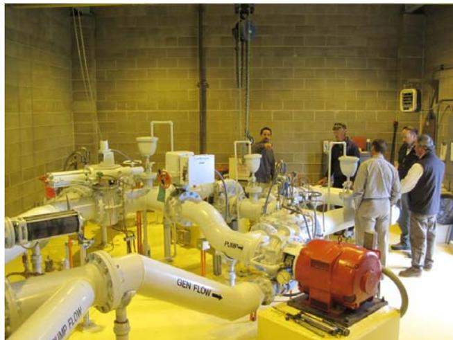
**Photo 14 - Kohler Hydro-Pump System Layout**
