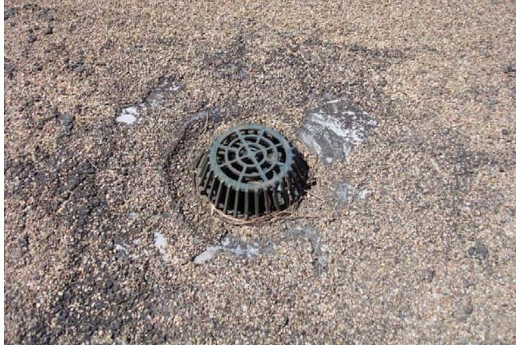
**Photo 18 - Chautauqua - Typical Drain Condition**
