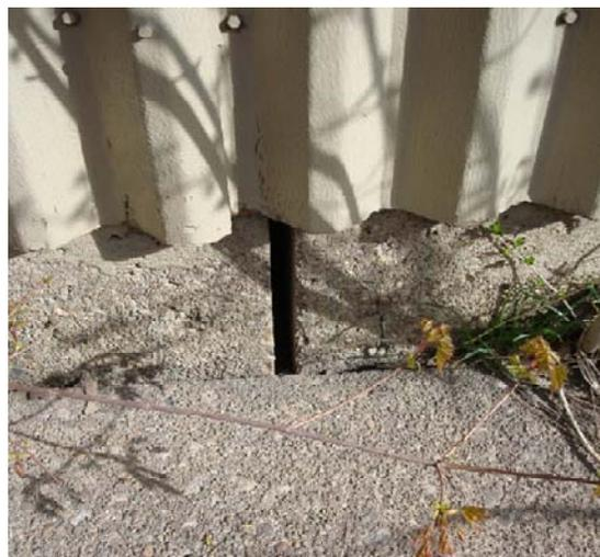
**Photo 10 - Kohler - Typical Movement Joint**
