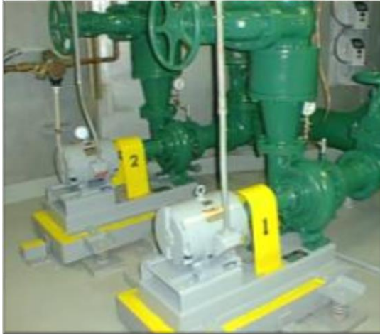
Photo 24 - Example of Variable Speed Drive Pool Pump
