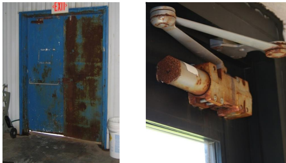
Photo 12 Examples of Results of Improper Painting in Aquatic Facilities
