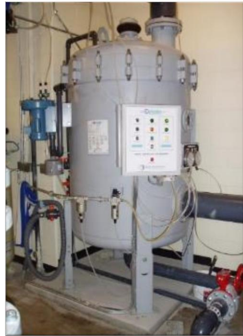
Photo 22 - Example of Regenerative Media Filter
