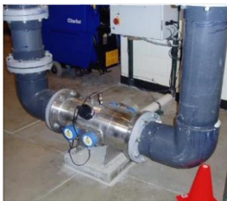
Photo 23 - Example of UV Sanitation System
