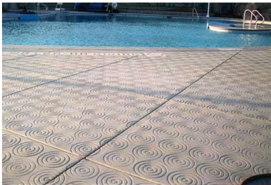
Photo 13 - Example of Safety Grooving of Concrete Pool Deck
