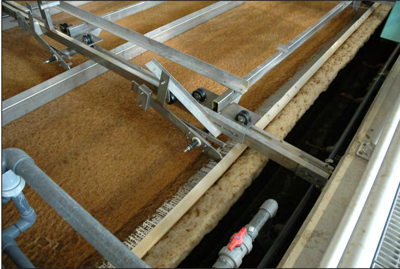
At the Boulder Reservoir Water Treatment Plant, residuals are scraped off of the water's surface. *Pettem photo, 2013.*
