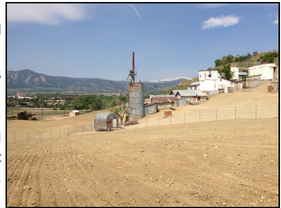
Valmont Butte Mill Site after the completion of the Voluntary Clean-up Program
