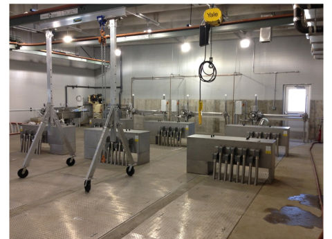
The completed UV Disinfection Improvements at the Wastewater Treatment Facility
