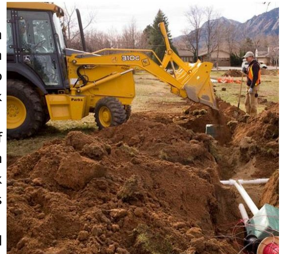
Urban Parks Irrigation Replacement underway
