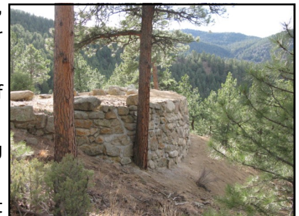
Chapman Drive Switchback after repairs
