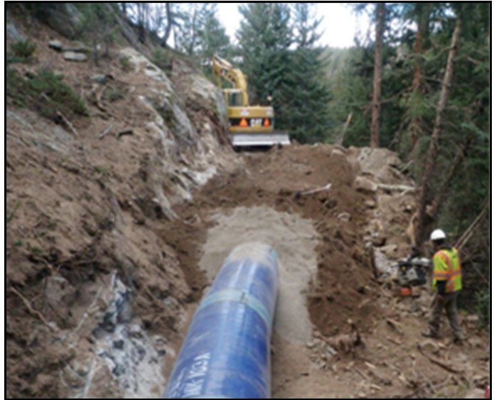
Repairs to the Barker Gravity Pipeline
