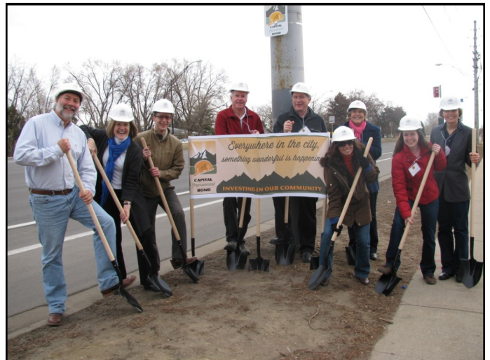
Groundbreaking of the first Capital Improvement Bond project in January 2012.
