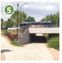
**Underpasses** and overpasses are facilities that are completely separated from car traffic by elevation.
